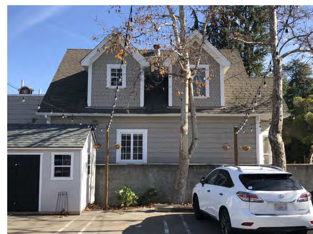
(P) EXISTING HOUSE (LOOKING UP EAST AT 12 MILES AVE FROM PROJECT SITE)
