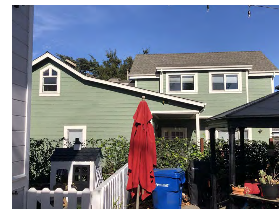
(P) EXISTING HOUSE (LOOKING UP NORTH AT 210 UNIVERSITY AVE FROM PROJECT SITE)
